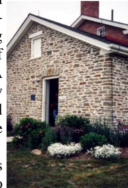
Rear entrance to the Dunton House
