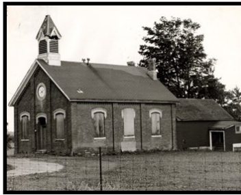
The schoolhouse pre-restoration
